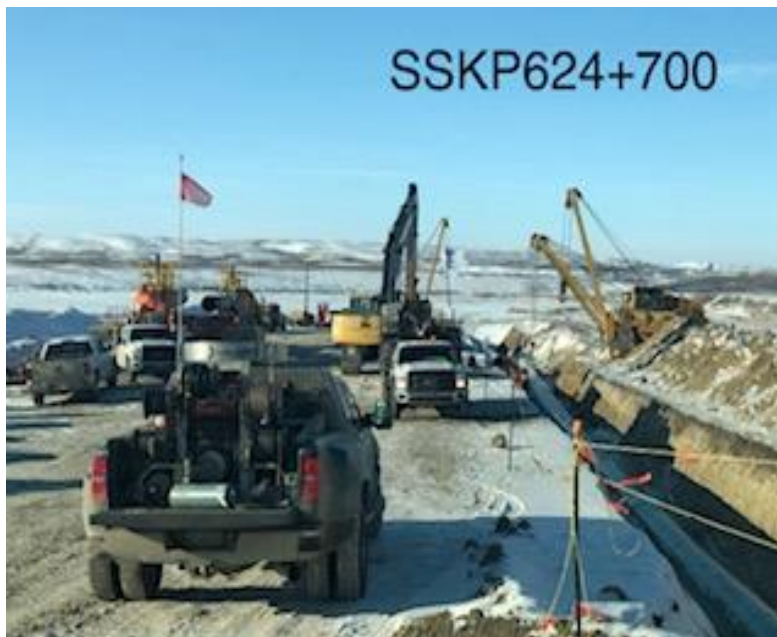
Chapleau Lake East side – tie in section
