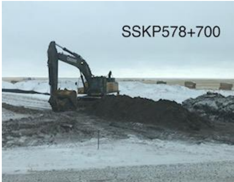
Ramp removal SF26 east
