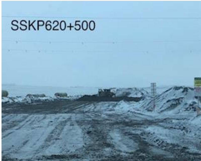
Machine Clean up continues
